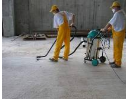
Cleaning of the surface
