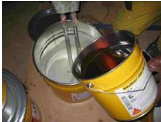
Mixing of Sikafloor-262 AS N
